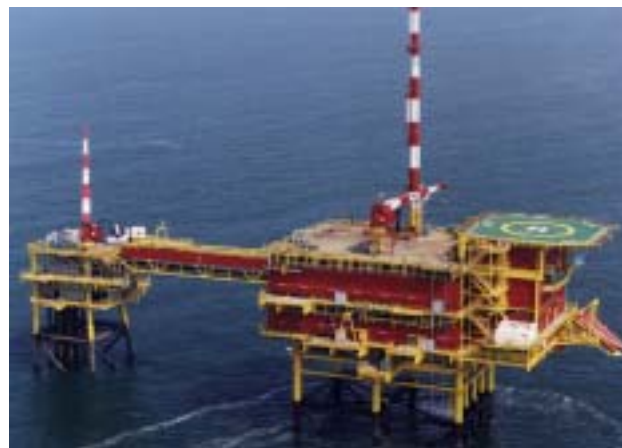
Wellhead and production platform at location L9
