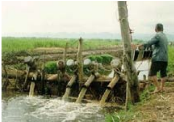
Water is pumped from Yilong Lake for irrigation
